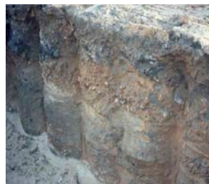
Tratamiento soil mixing tipo muro.
